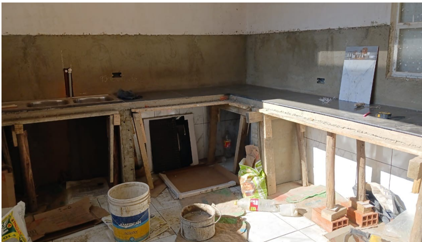
Work on the kitchen at Tabita House which MWiB is supporting
